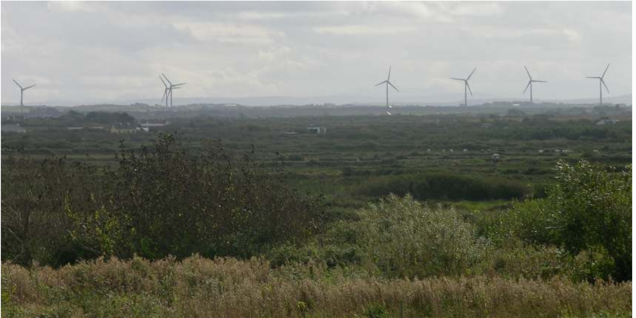
Moanmore Wind Farm, Clare / Enercon 7xE-70 2MW
